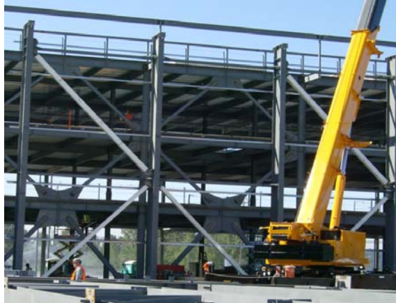
Fig. 16. Braces (white, foreground) installed in single diagonal configuration
