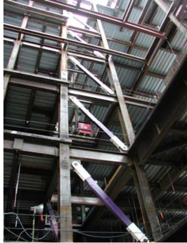
Fig. 7. Star Seismic PowerCat braces used as single diagonals
