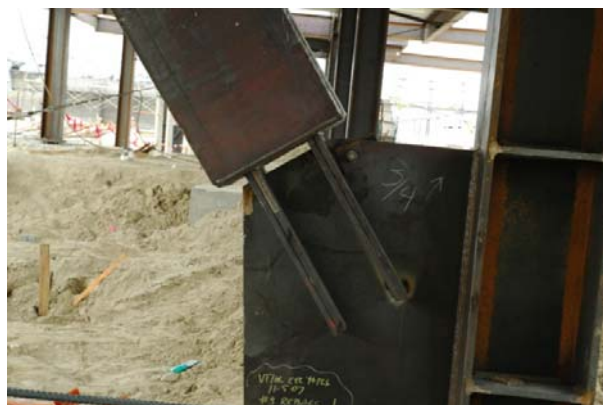
Fig. 14. Welded connection detail
