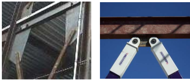
Fig. 8. Conventional and BRB connection
