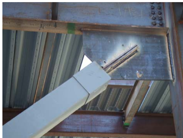
Fig. 10. Welded end connection of the braces
