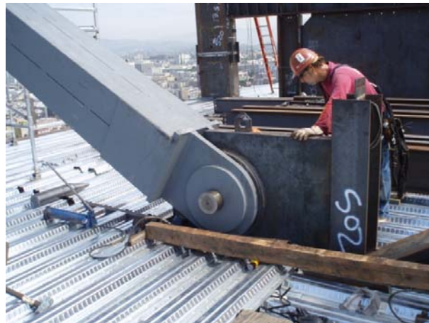
Fig. 9. Pinned connection
